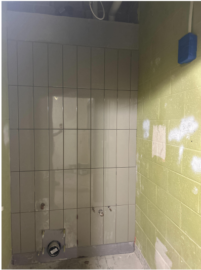
Installing ceramic tiling in restrooms on level 1.
