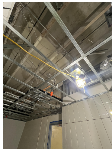
Installing ceiling grip in the administration office on level 2.
